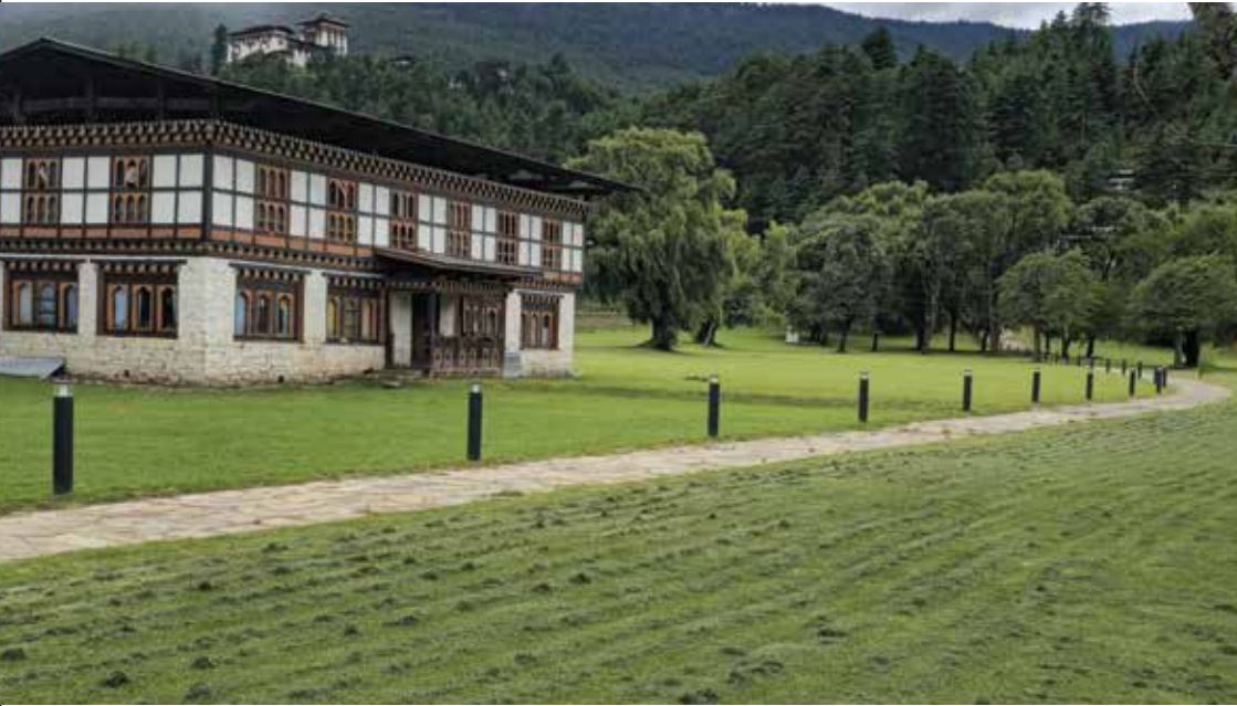
WANG PALACE, BUMTHANG, BHUTAN
